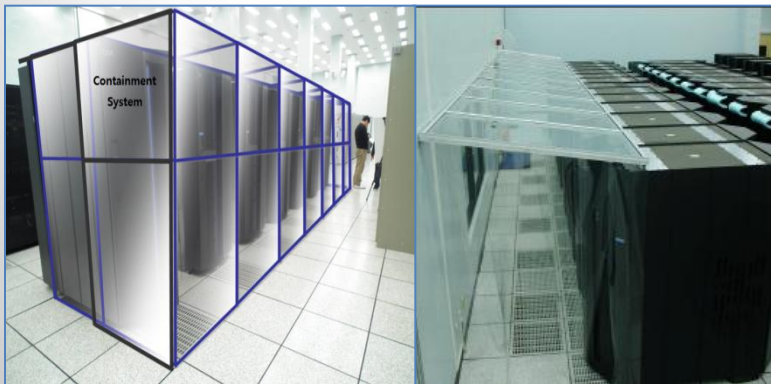
Cold aisle containment
